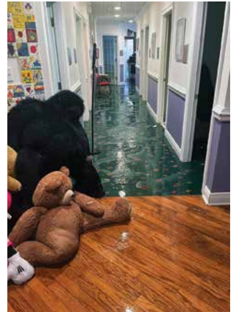
ECCAC's Niceville Center was severely damaged when their building's sprinkler system put out a fire that caused significant subsequent water damage.
